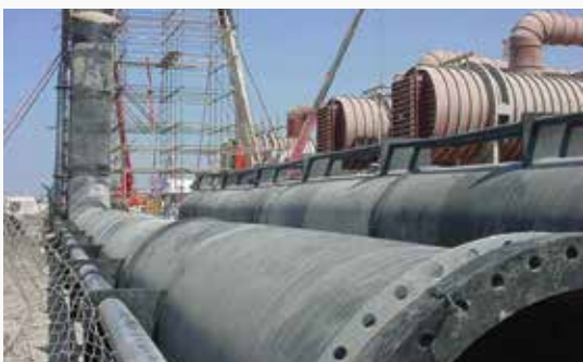
NIC HDPE Corrugated Pipes with flanged connection for sea water intake project in UAE
