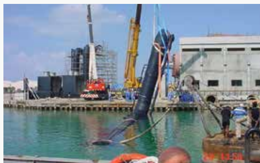
NIC HDPE Corrugated Pipes for sea water intake project in UAE
