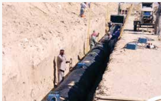
NIC HDPE Corrugated Pipes for Storm Water with electro-fusion connection at project in Kuwait
